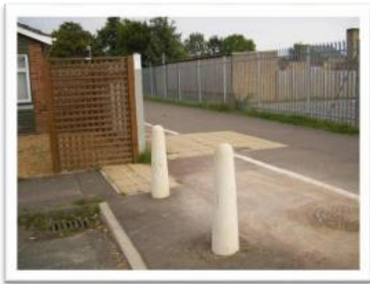
Alfred Cope Road / Cycle Path
